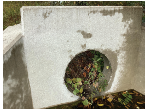
LOT 57 Precast Concrete Spillway
